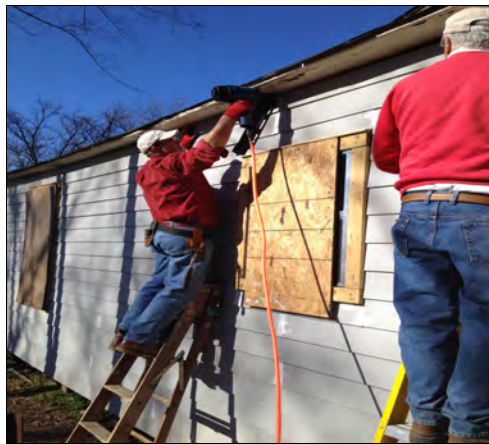
Concrete-based HardiePlank Lap Siding installed over all new sheathing.
