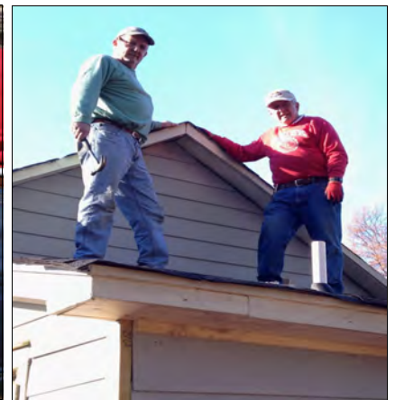
The last piece of HardiePlank
