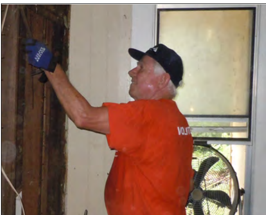
Inside and out, volunteers stripped the house to the studs, replaced rotten and termite-infested wood and then started rebuilding.
